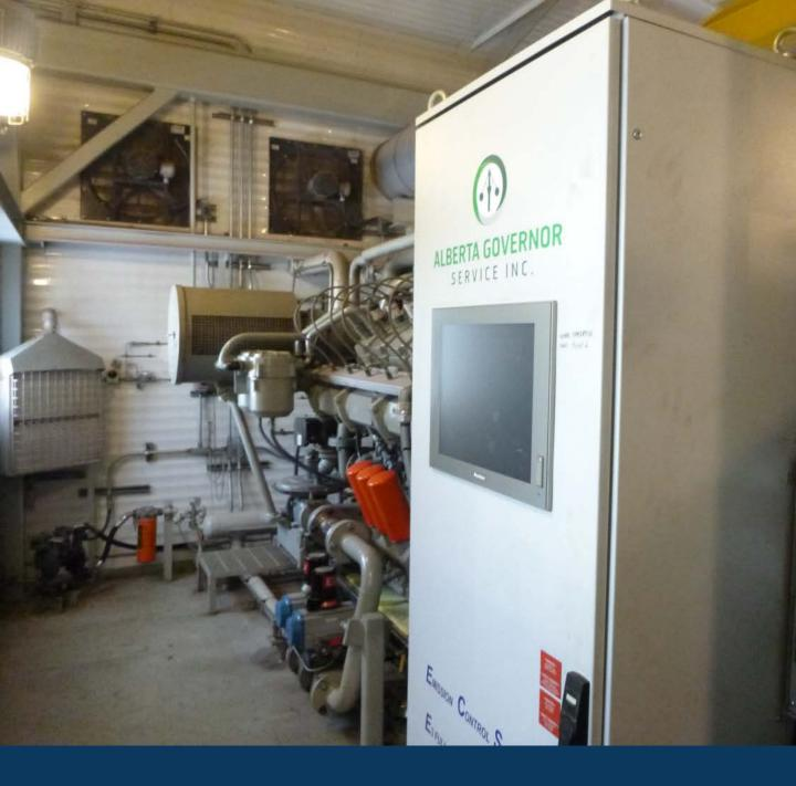
As New Condition – This 4MW power plant is comprised of two buildings each housing two (2x) 1250KVA generators and driven by Waukesha 16V APG1000 Series engines (designed for power generation specifically) and operate at ~40% efficiency. These generators are not only low hour, but have been meticulously maintained and operated – even as the owner waits for new, smaller diesel units to arrive, these generators are still fired up and run for one hour per month.
