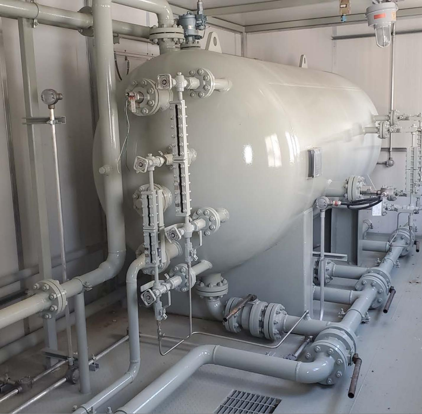
Designed to work with 150HP Jet pump packages (sold separately), these separators are designed two phase, but the designers really had a fascination with level gauges, and as such you will have amazing optics on what is happening inside the vessel. There are 5 available, 2 are new – 3 are used and in great condition still. All of them are located in an easy access yard in Grande Prairie, Alberta for easy removal and transport to your site.
