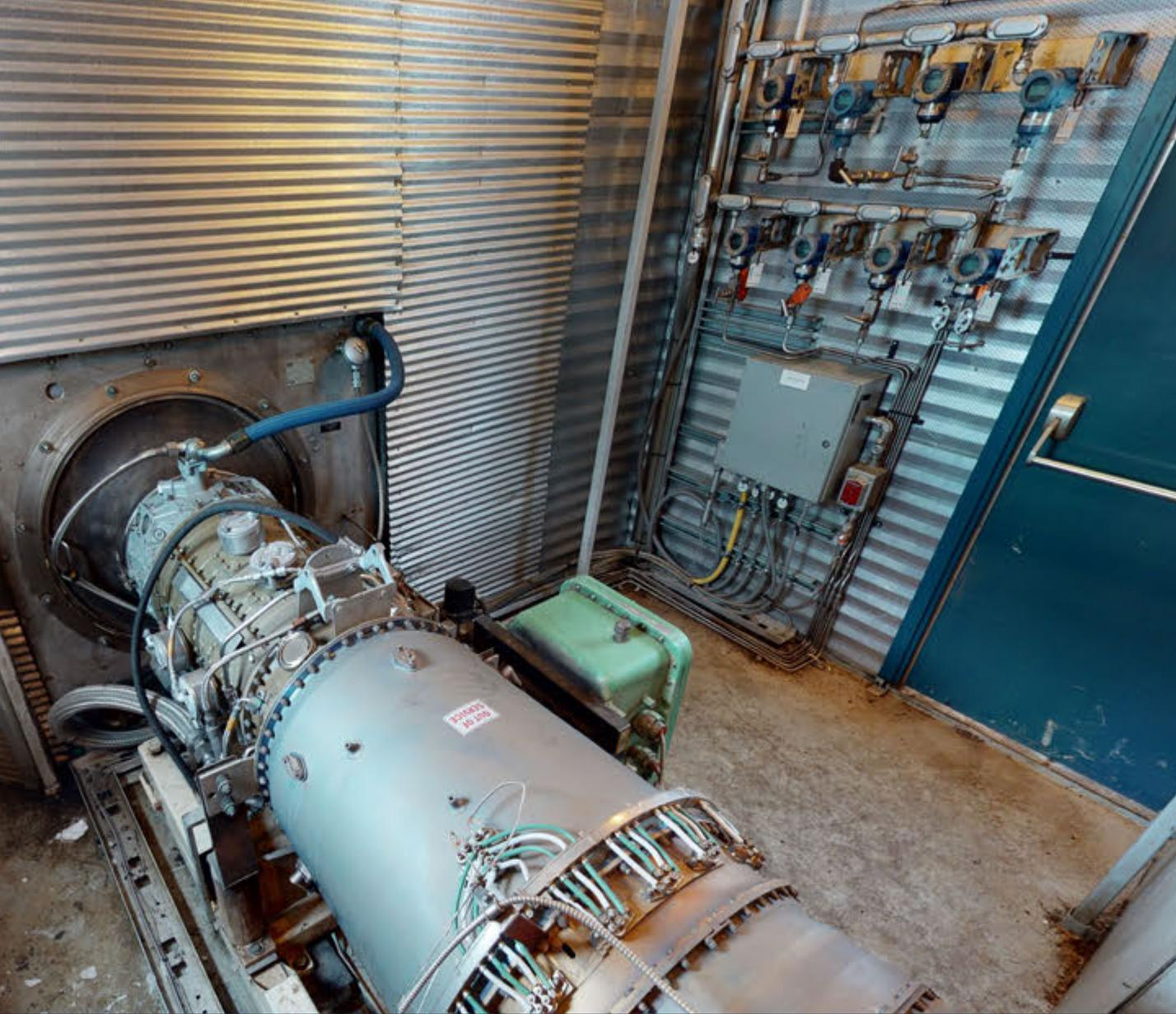
Sitting in Central AB, these two Allison gas turbine generator packages are each capable of producing 2.5 MW of power. The system comes with grid connect equipment, as well as a thermal oil heat recovery system.
