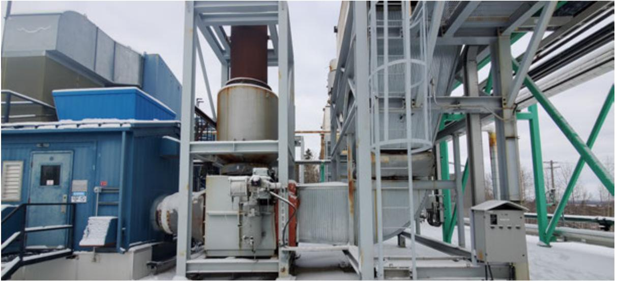
*Designed for hot oil – operated at 300°C. Each turbine is equipped with a waste heat recovery thermal oil heater tied into a common 48" surge vessel c/w dual centrifugal pumps on a skid.*
